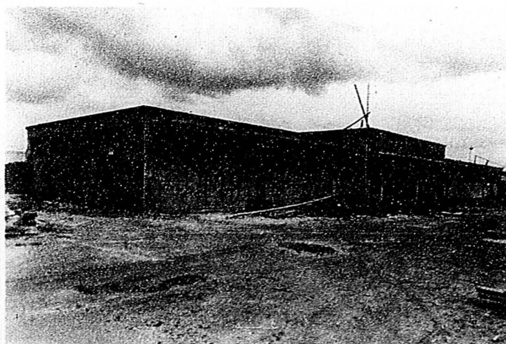
CONSTRUCTION AGENCY OKINAWA ENGINEER DISTRICT LINE ITEM NR AND PROJECT DESCRIPTION 1019 Guard House LOCATION Fusuma Air Base CONTRACTOR Zenitaka Gumi % PROJECT COMPLETED 50% CONSTRUCTION DIRECTIVE OKI-417-56-1 CONTRACT NR FEC- 505 PHOTO DESCRIPTION The Guard House No. C at Fusuma Air Base showing all concrete and most of block work complete. PHOTO NR 5055-2 DATE 6 Jan. 1955
