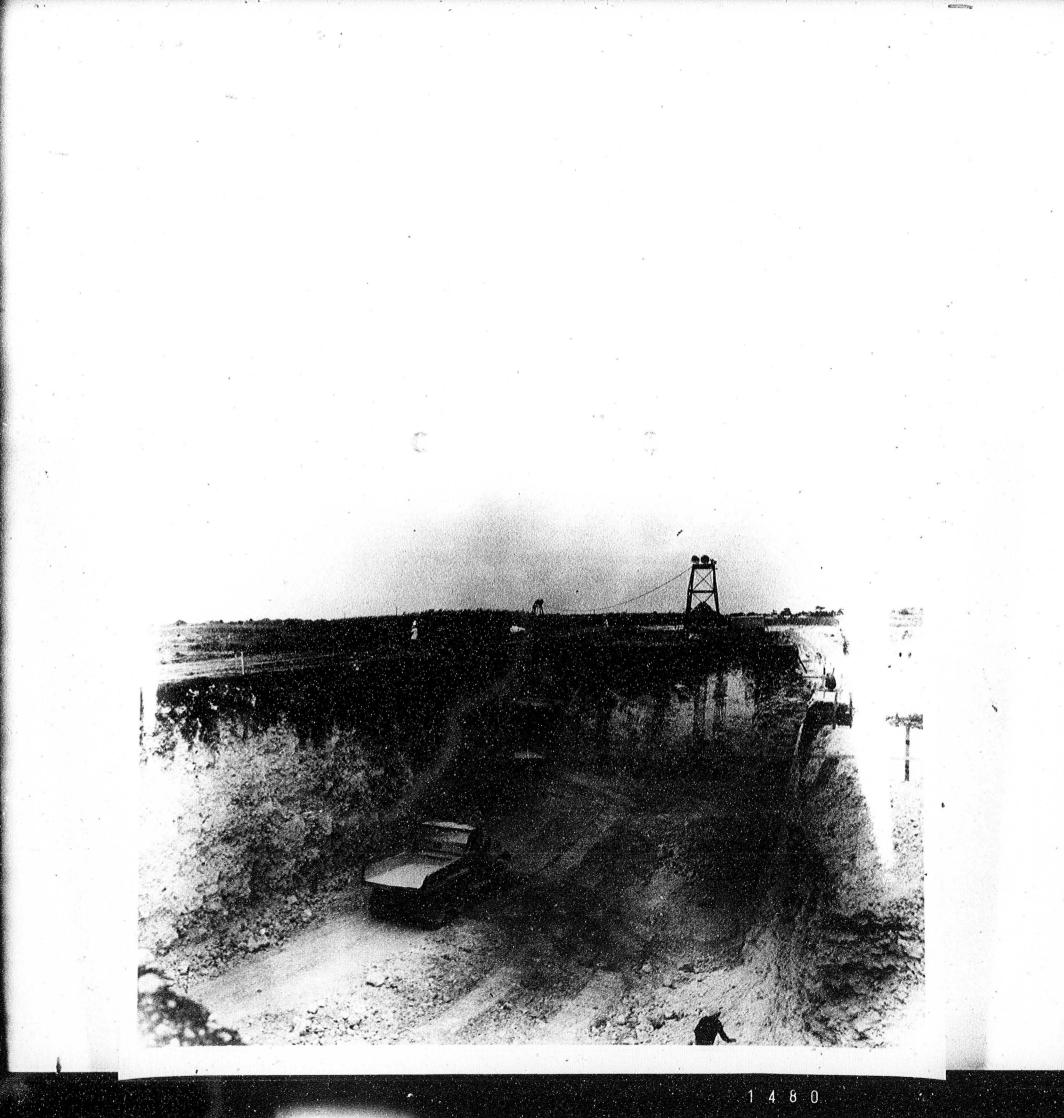
MACE SITE #2 AT WHITE BEACH AT 90 PER CENT STAGE OF COMPLETION FOR PHASE ONE--EXCAVATION--AT THE TIME THIS PICTURE WAS TAKEN ON 1 JUNE 1960. ITS DEPTH IS 29 FEET. THE CONTRACTOR FOR PHASE ONE WAS THE M-G CONSTRUCTION COMPANY, AN AMERICAN
